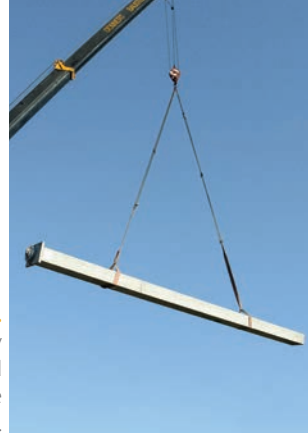
Prefabricated Chimney. The ATMOS will be already completely prefabricated for the full height of the building.
